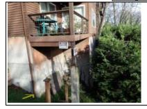
Controlling roof drainage is critical to protect the housewall from water/moisture problems and damage, and preventing excessive surface water at the foundation wall. This may be controlled as easy as cleaning the gutter system; replacing all rusted/leaking gutters/downspouts; making sure all connections are water-tight and made appropriately; and that all gutter system components have been installed.
