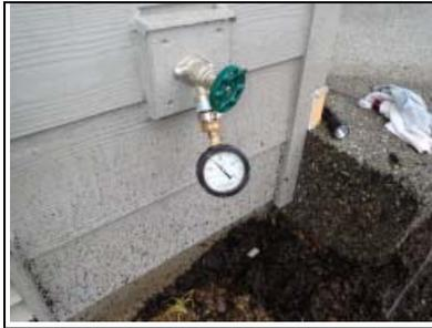
**Potable Water Temperature:** Temperature Settings; 120F degrees.
