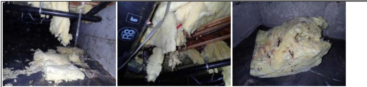
**Conducive Conditions:** High moisture conditions observed during inspection- potential for wood-decay rot, molds/mildew and rodent and insect infestation. Posts are at/below grade level and are sitting in the water through the middle of the house.
