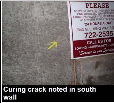
Curing crack noted in south wall
