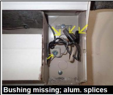
Bushing missing; alum. splices
