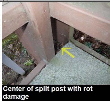
**Center of split post with rot damage**
