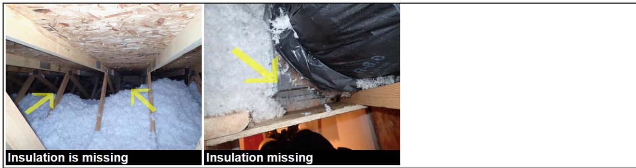
Insulation R-Factors: The effectiveness of insulation is rated by its ability to slow heat transfer, as measured by its R-factor. Because the R-factor varies according to the density and other properties of a material, it is also related to thickness. Typically, the deeper/thicker the insulation, the higher the R-value. In older homes, you may find minimal amounts of insulation, or you may also find multiple layers of different types of insulation, where they were added over the years.
