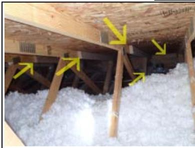
Roofs are constructed either with rafters (conventional stick-framed), engineered trusses (most common for newer construction), open beams or some combination of these types and styles. Stick-framed roofs are usually made with dimensional lumber (2x material), but may also use composite/engineered materials. Stick-framed is still used in many cases because it is the most flexible roof framing system. This is often found in complicated roofing systems, vaulted ceiling and low pitched roofing.
