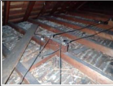
Insulation R-Factors: The effectiveness of insulation is rated by its ability to slow heat transfer, as measured by its R-factor. Because the R-factor varies according to the density and other properties of a material, it is also related to thickness. Typically, the deeper/thicker the insulation, the higher the R-value. In older homes, you may find minimal amounts of insulation, or you may also find multiple layers of different types of insulation, where they were added over the years.
